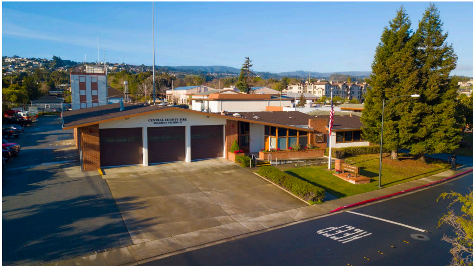
Fire Station 37 511 Magnolia Avenue Millbrae, CA 94030
